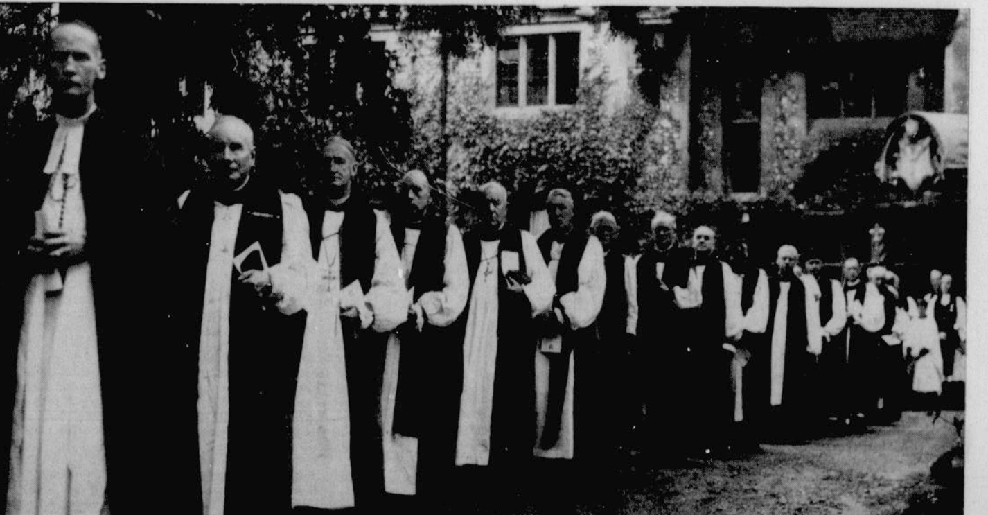
Twenty years ago the 1948 Lambeth Conference opened at Canterbury. Australian archbishops and bishops moved in procession from the Old Palace to the Cathedral.
